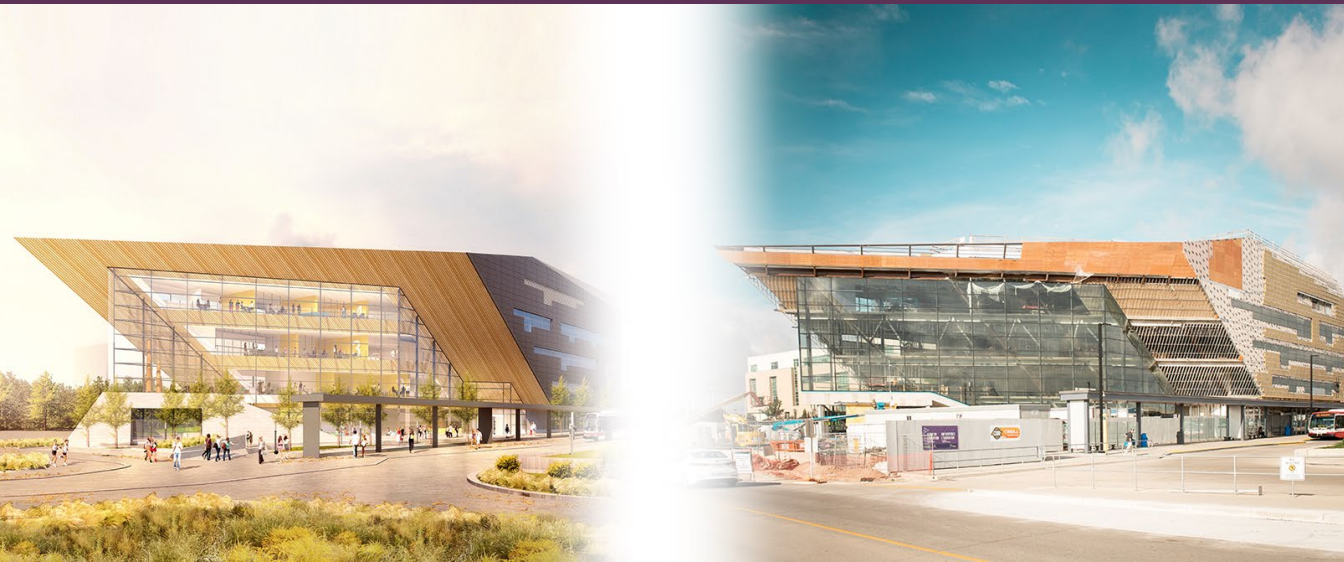
The Barrett Centre for Technology Innovation is slated for completion in early 2019. Rendering of the completed Barrett CTI (left), construction progress as of August 2018 (right).
